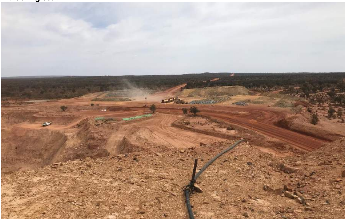
ROM Looking North.
